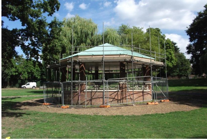
Bandstand Restoration Works in Raphael Park
